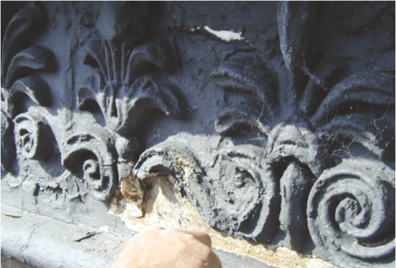
Detail of Plaster before renovation
