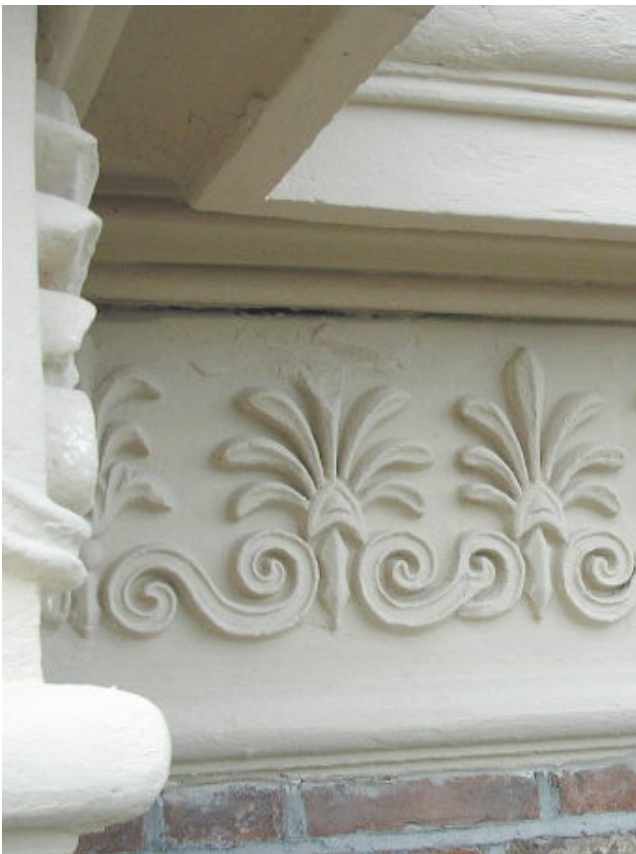
Plaster Frieze after renovation (left)
