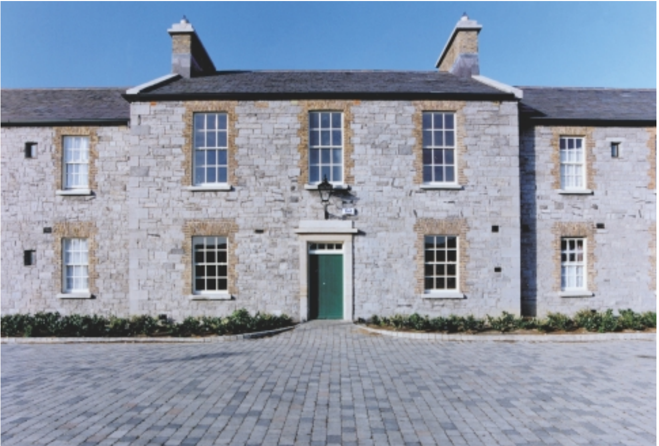
Top - Buildings converted to residential use Beggar's Bush
