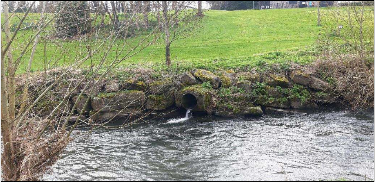
Figure 2-6 Outfall within Tolka Valley Pitch & Putt Course
