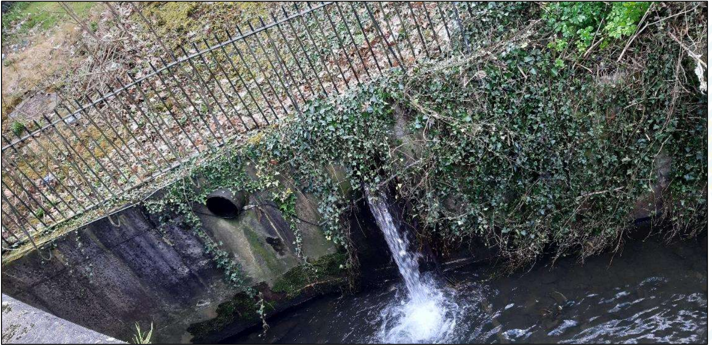
Figure 2-5 Outfall pair at Tolka Bridge, Note the outfall from the 750mm culvert to the right of photo with flow present
