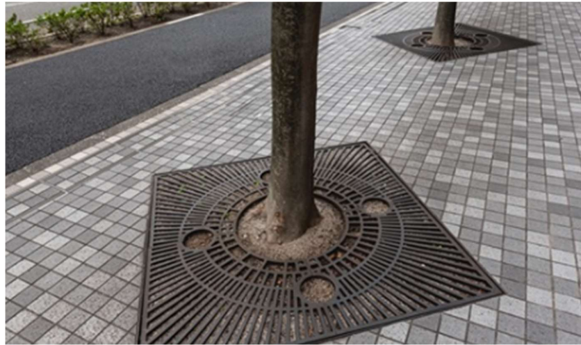
Figure B-5 Tree Pit (Source: GCL Products)
