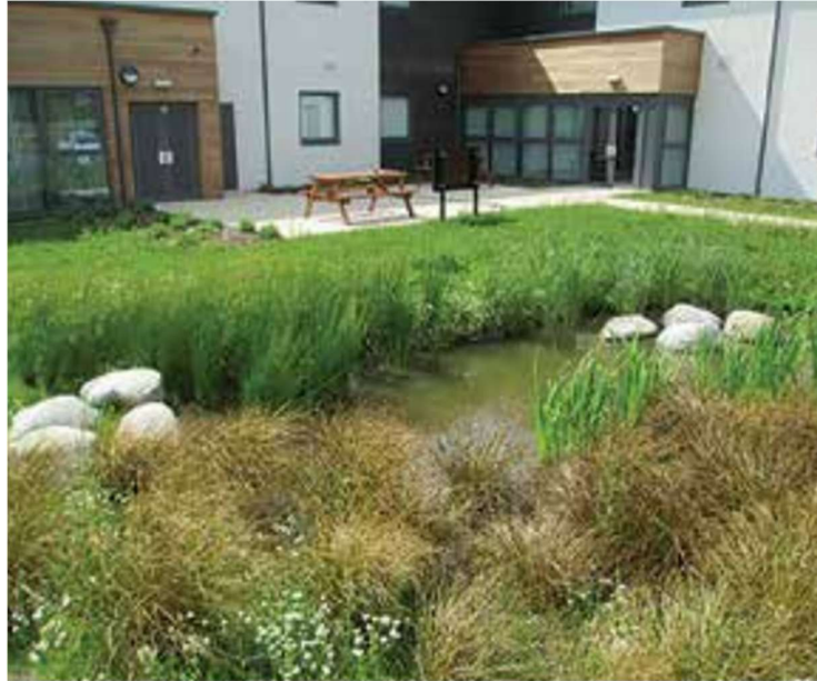
Figure B-3 Raingarden (Source CIRIA Manual C753)
