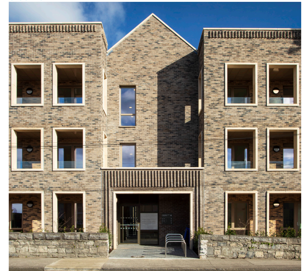
Figure 5.4: Springvale Groove. DCC City Architects. Image by Niall O'Connell.
