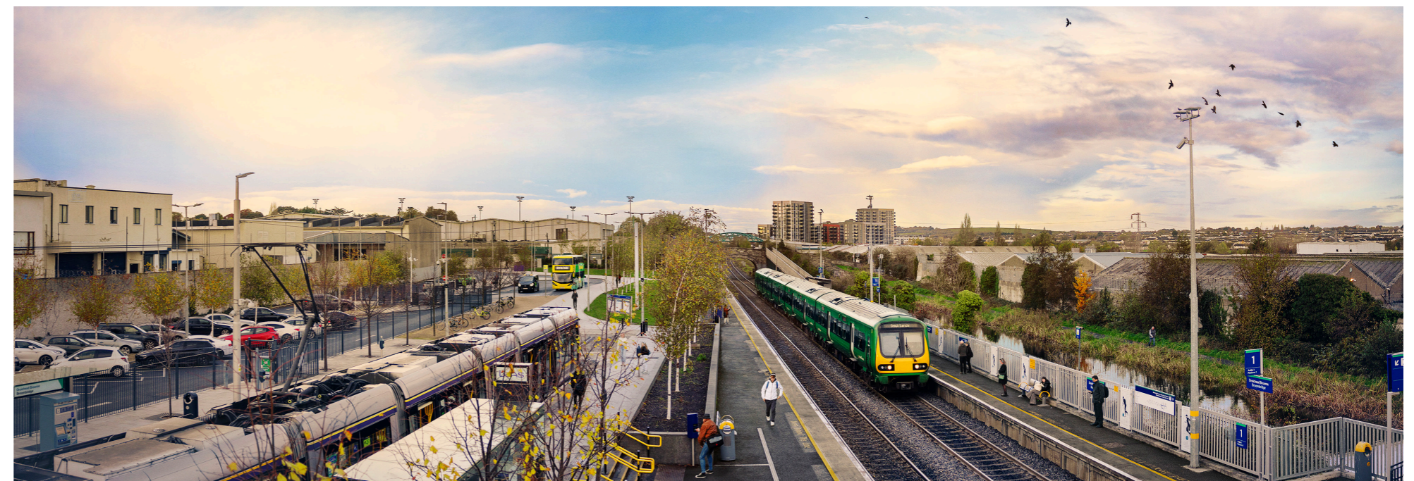
Figure 3.11: Broombridge transport interchange. Image by National Transport Authority.
