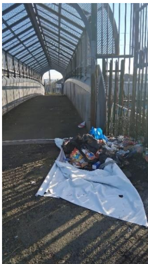
Irish Rail foot bridge, Cherry Orchard
