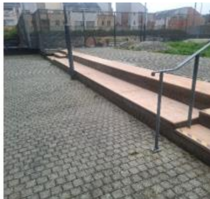
New timber installed on the seating and steps outside F2.
