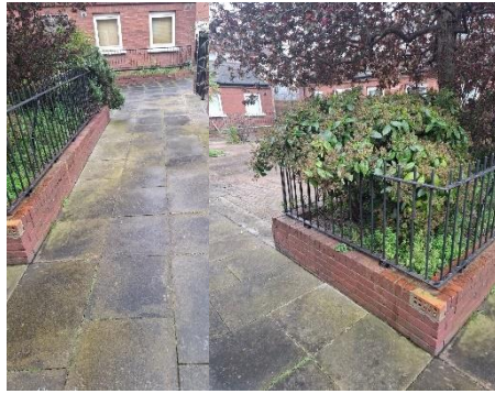
Weeding and clearing of vegetation within the complex. (before and after).
