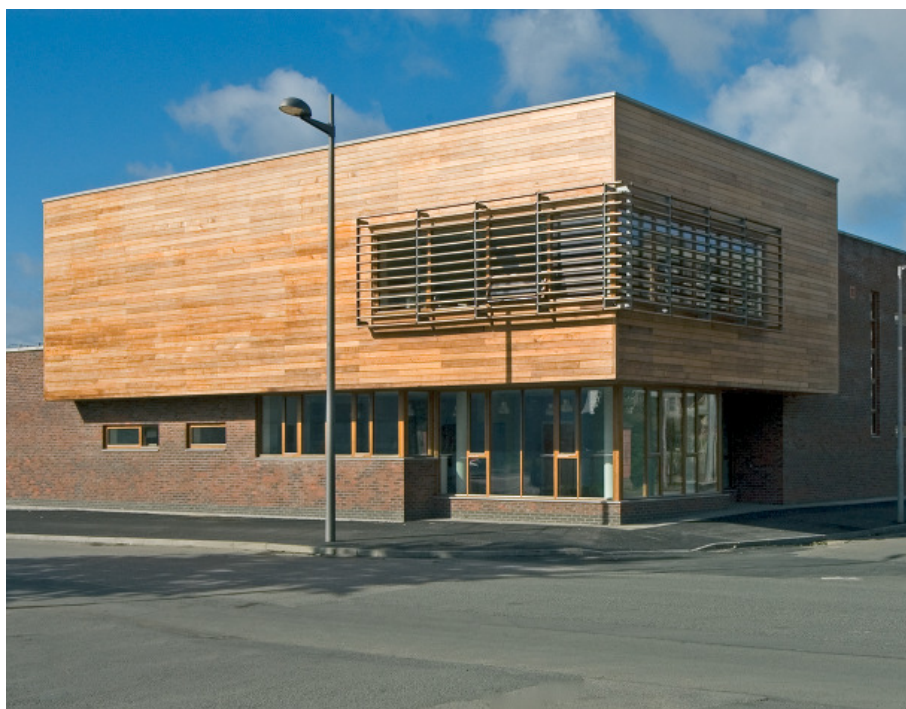
The Reco, youth facilities building
