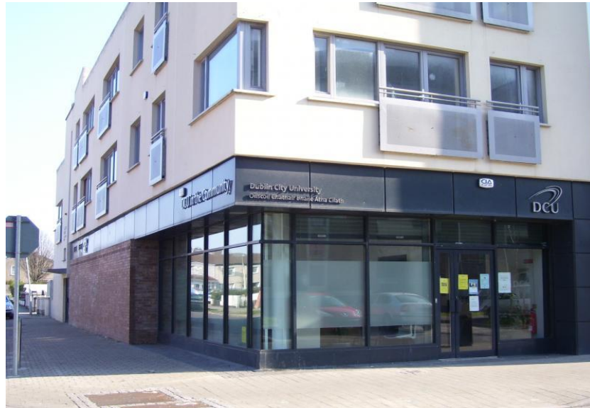
Figure 1 – University College Dublin – Ballymun Office
