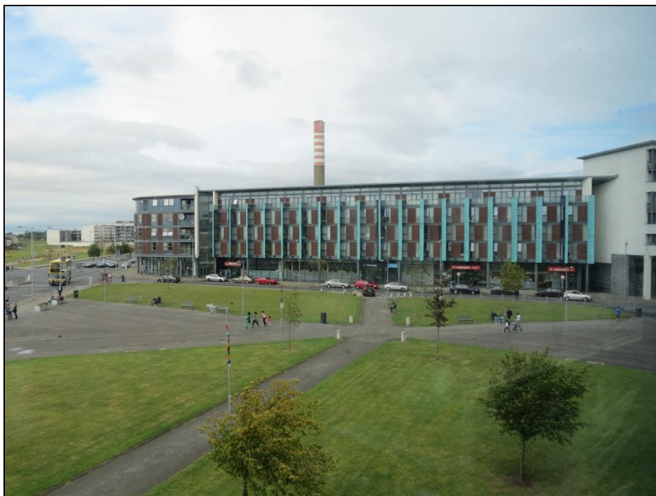
Fig 7.5 Ballymun Plaza in front of Civic Centre (Axis Theatre)
