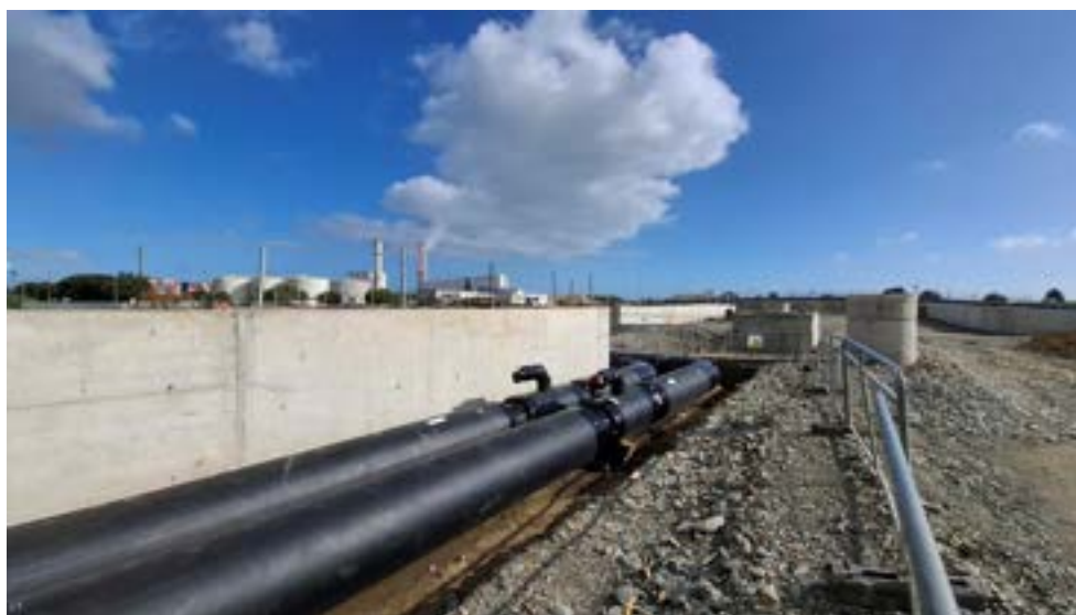
Hot water piping network installed at Irish Glass Bottle Site
