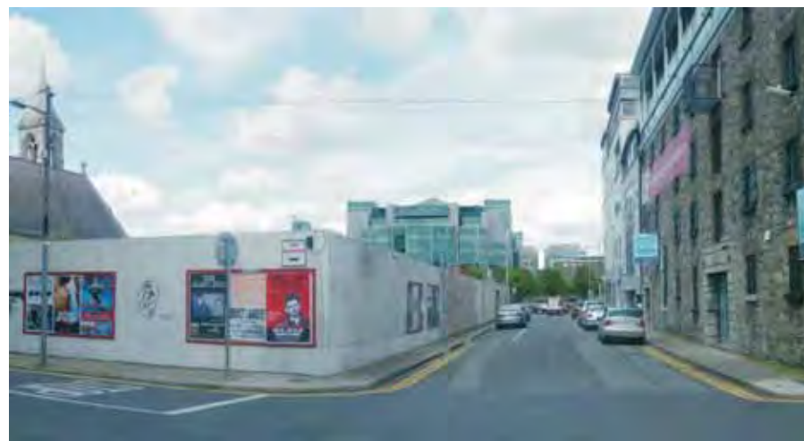
Princes Street South - Existing Situation
