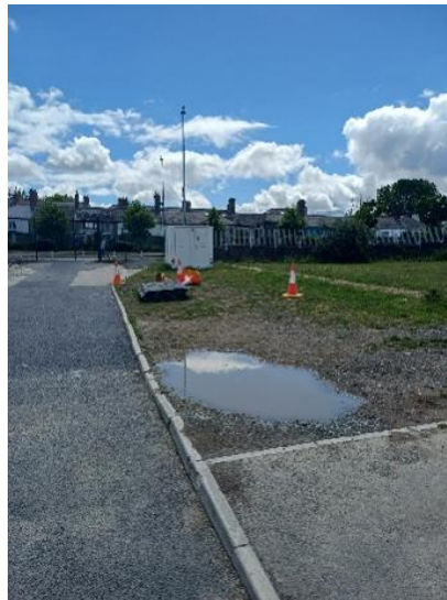
Site of completed roadworks undertaken to relocate gas network pipes.
