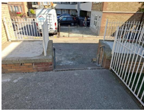
Planters at Blocks B/C filled in with concrete (before and after)
