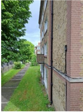
Cables tidied outside Oliver Bond House (before and after)
