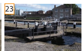
23 BRITAIN QUAY / HANOVER QUAY (RPS 987)
