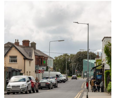
Lack of greening, few resting spots
