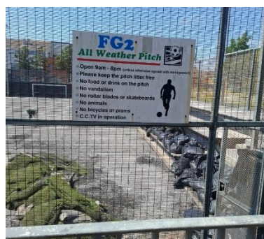
The pitch at the F2 Centre is currently undergoing resurfacing works.
