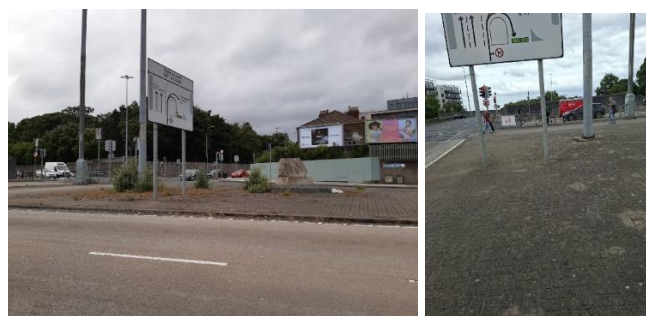
Traffic Island SCR /Islandbridge
