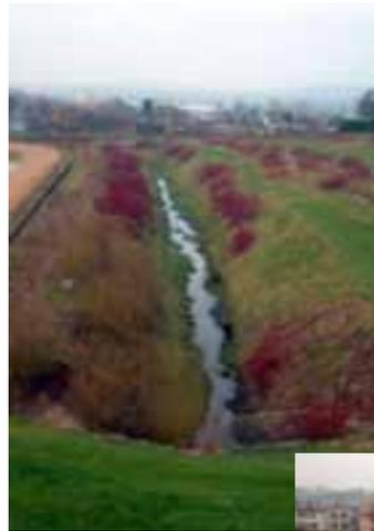
*Large swale receives motorway drainage.*
