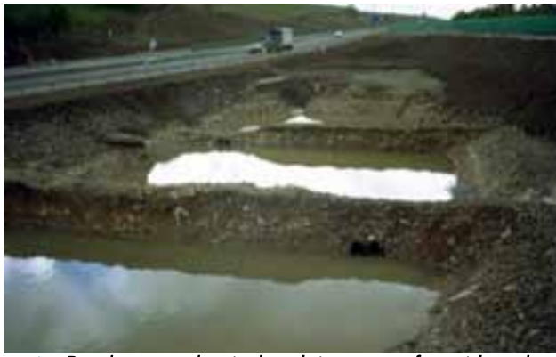
Settlement lagoons installed during construction; retained for permanent use.
