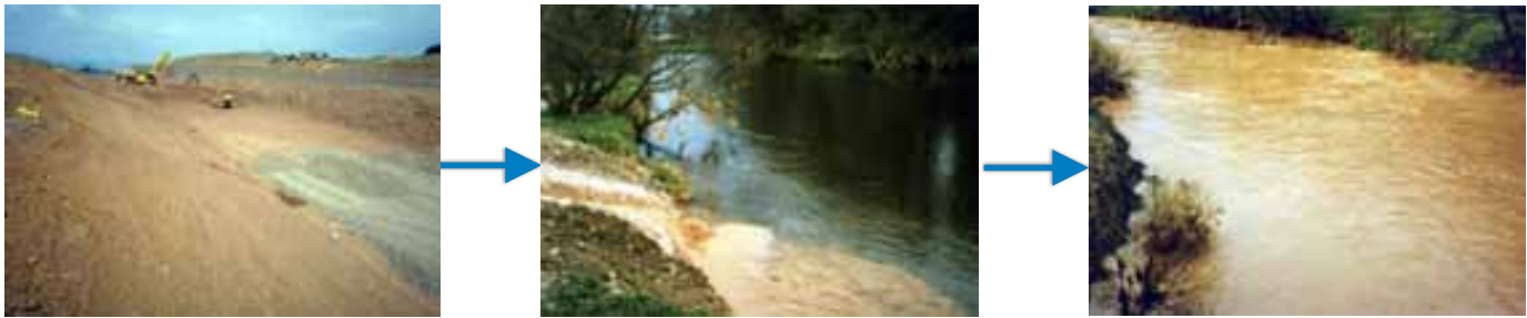
M74 construction led to pollution of the River Annan which spread rapidly.
