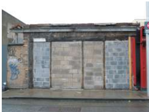
Figure 1: No. 6 Post demolition Photo: BAR Photographic Survey: 26/03/12
