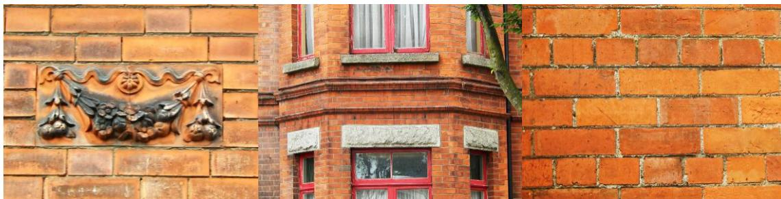
Walls are the main structural fabric of any building. Every effort should be made to retain or re-use original facing brickwork, vitrified brickwork, stonework or render styles. Alterations or repairs to external walls should respect the original material and endeavour to match it in appearance.
