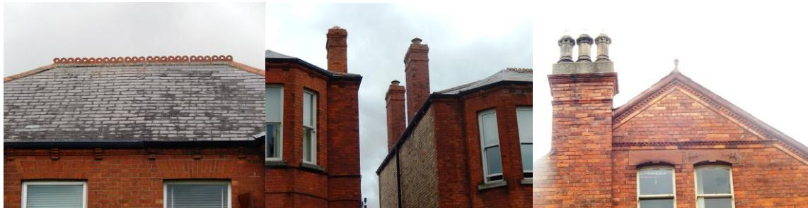
The roof is often an important feature of a historic building that can make a significant contribution to the character of an area. Historic roof materials and features such as chimneystacks, chimneypots, natural slates, dormers, roof lights, as well as details such as decorative ridge tiles and finials all form an integral part of the character of the building and should be retained.
