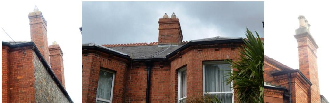
Original rainwater goods are an integral part of the design and character of an historic building. They will normally be cast iron, which if properly maintained should last many years longer than replacement plastic goods. Cast iron gutters, down pipes and hopper heads etc should be retained wherever possible. Plastic rainwater goods are not considered appropriate on buildings where cast iron has been previously used.
