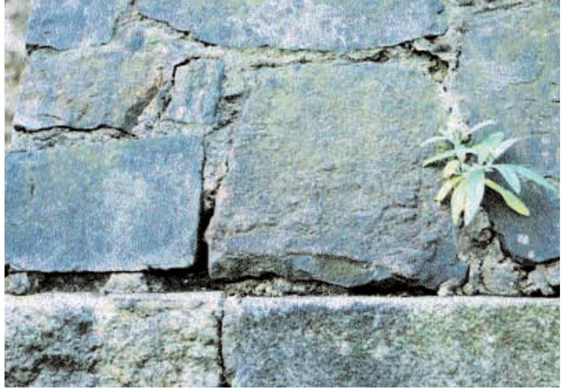
Plate 5 Missing stones in the buttress of the City Wall on Cook Street.
