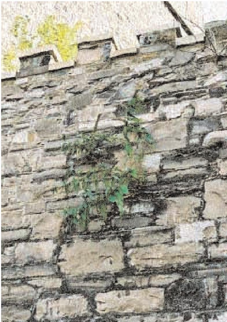
**Plate 8** Sulphation of mortar.
