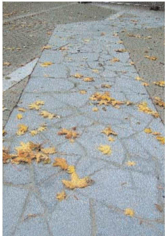
Plate 13 The existing pavement treatment marking the line of the wall below ground at the Civic Offices.
