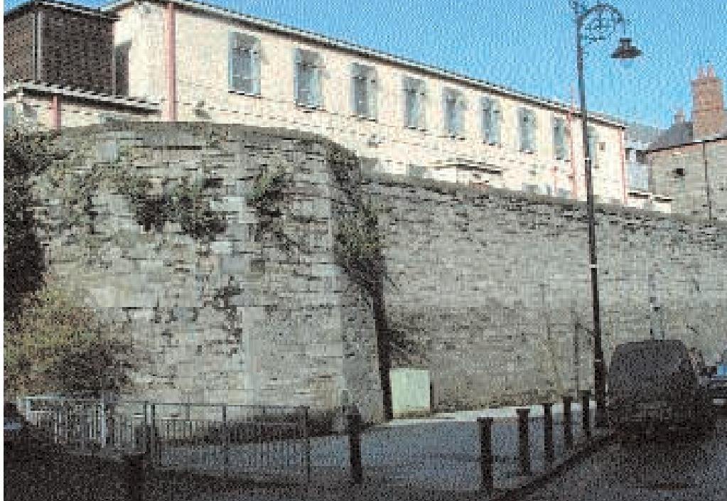
**Plate 26** Original masonry and later interventions at Ship Street Little, near Werburgh Street.
