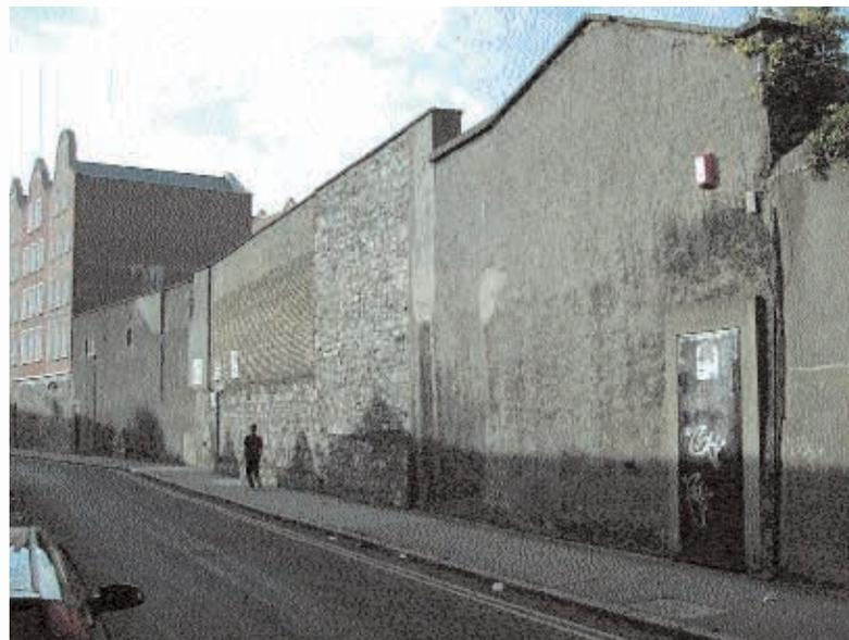
**Plate 38** Wall along, Lamb Alley incorporating original City Wall fabric and thought to follow its original line. Note the stringcourse.
