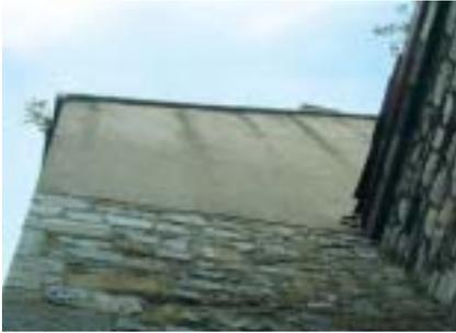
**Fig. 7.14** Section of dense cement render on the east gable with some cement pointing under – probably date to early 20th century construction of apse.
