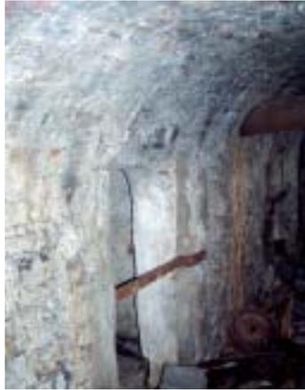
**Fig. 7.30** Crypt interior – view to crypt entrance with corroded metal bar protecting entrance.
