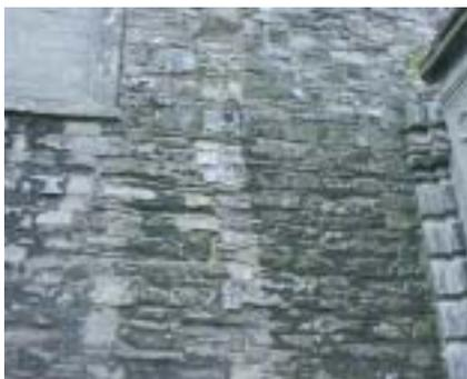
**Fig. 5.7** The church is constructed of rough-coursed calp stone.
