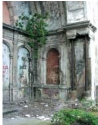
**Fig. 7.17** View of south double pilaster where iron column structure has been completely exposed.
