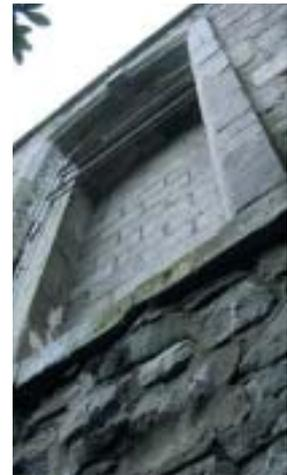
Limestone (Dublin calp) window surround with some surviving iron glazing bars in a corroded condition. Windows have been blocked up crudely for security.
