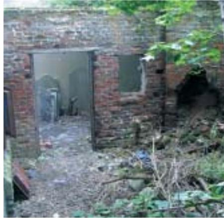
**Fig. 7.20** *Surviving brick shell of original vestry with corner fireplace, and timber lintels to door and window opes surviving. Note tombstones stacked against boundary wall in the background.*
