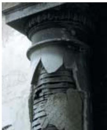
**Fig. 5.35** The lath and plaster columns enclose structural iron stanchions.
