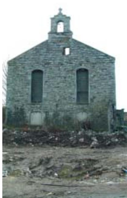
**Fig. 5.19** *Exterior view of western gable. Note the random rubble on the lower portion of the wall and the coursed block-dressed stone above the eaves.*
