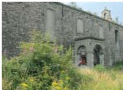
**Fig. 9.4** Front (northern) area May 2003 showing extensive growth and build up of ground level.
