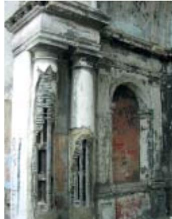
**Fig. 7.16** Detail of chancel showing construction of cast iron column structure with lath and plaster covering.
