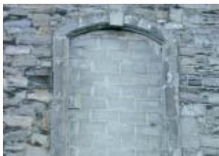
**Fig. 7.24** Concrete blocks to window ope on north façade.
