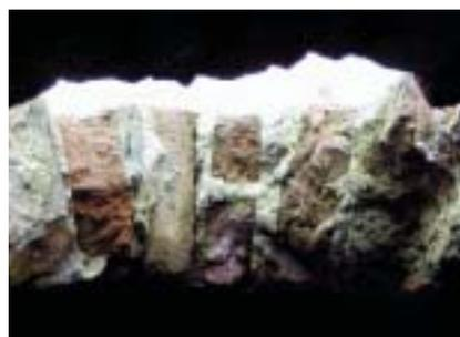
**Fig. 7.27** View through ope in floor showing brick vault construction to crypts.
