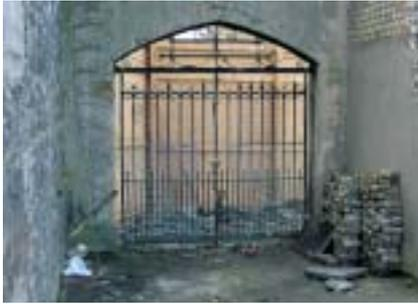
**Fig. 7.9** Inner, rendered face of Newmarket entrance gate prior to temporary removal of gate and propping with concrete blockwork.
