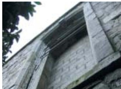
**Fig. 7.25** Window ope on south façade are blocked up on the inside with reveal and surviving iron glazing bars exposed to external.
