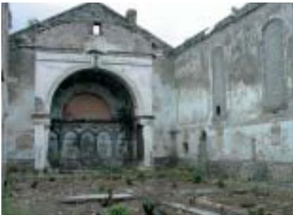
**Fig. 7.15** Internal view of church, showing considerable amount of internal plaster surviving, the east end chancel and the scar where the dado panelling was removed.
