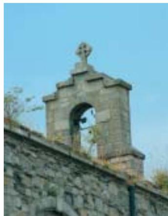
Some structural consolidation is required, particularly at wall tops, where weathering and vegetation will have desta-
