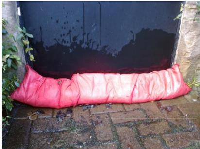
These are modern alternatives to conventional sandbags. They are lightweight, easily stored and deployed, and some are re-usable. They are also significantly more water-proof than conventional sandbags. They contain a special polymer that is activated by immersing in water for a few minutes and they can be moulded to fit the location where they are to be used. However, they tend to have a shelf life of above 5 years (even if they were never used) – homeowners should check this before purchasing
