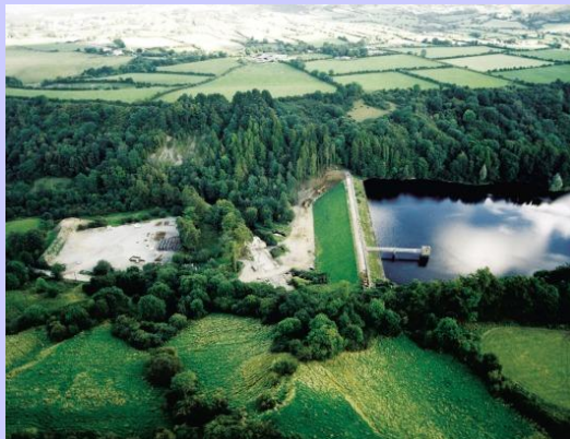
Fig. 18: Water turbine (90 kW) at Roundwood Waterworks provides 100% of the power requirement for the works
