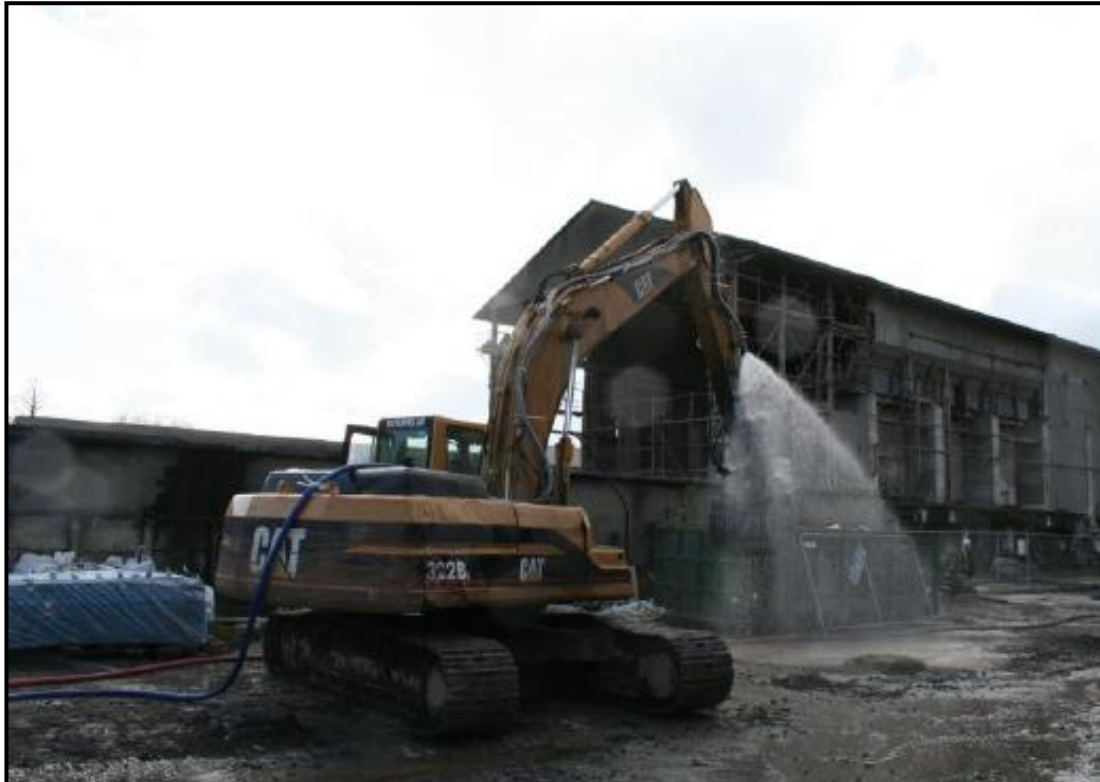
Photo 11.1: Demolition Excavator fitted with high power water hose on boom
